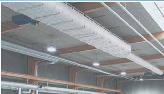
*Rectangular ducts are typically created using internal membranes for structural integrity, and support hoops may be used on all four sides. This ensures that the duct keeps its profile when the air is turned on, despite the natural pressure toward bulging.*
